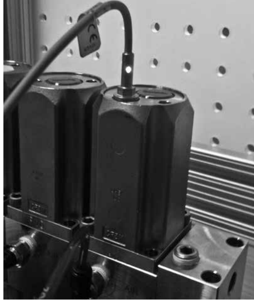
Fig 19 Valve Indicator Light
