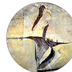
Excessive Cover Damage
