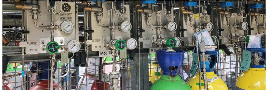
A major British chemical company uses various specialty gases to perform research and development functions. Many of these gases can pose a significant risk to workers if they are not safely contained, making leak-tight gas distribution and handling throughout more than 200 gas lines a top priority. The company took advantage of the Swagelok gas distribution program to enhance the safety of its system and realize new efficiencies.
