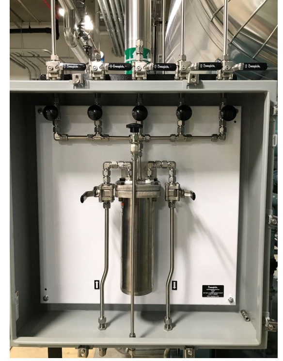
Condensate Sampling Panel
