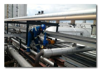
On October 10th, 2017, we conducted our first on-site Compressed Air Survey at where we tested 15,000+ fittings over the span of **8 days**. Of the 15,000+ fittings tested, **5.4% leaked**, which amounted to **817 leak points** detected at the AltaGas site. They received a detailed report on our findings, which prioritized leaks by severity, to assist in the repair and reduction of leak points, and the quantified cost of avoidance of the associated emissions.
