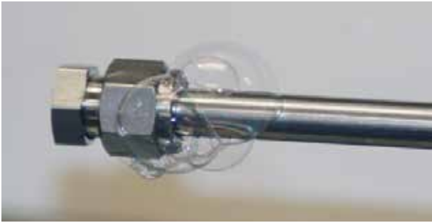
Figure 10-8 Larger leak displays large bubbles.
