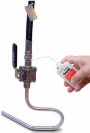
Figure 7-3 Snoop leak test.
